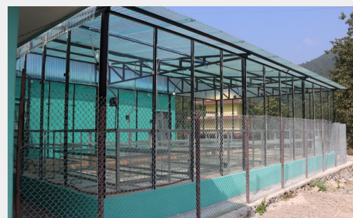
Newly built solar drying facility
